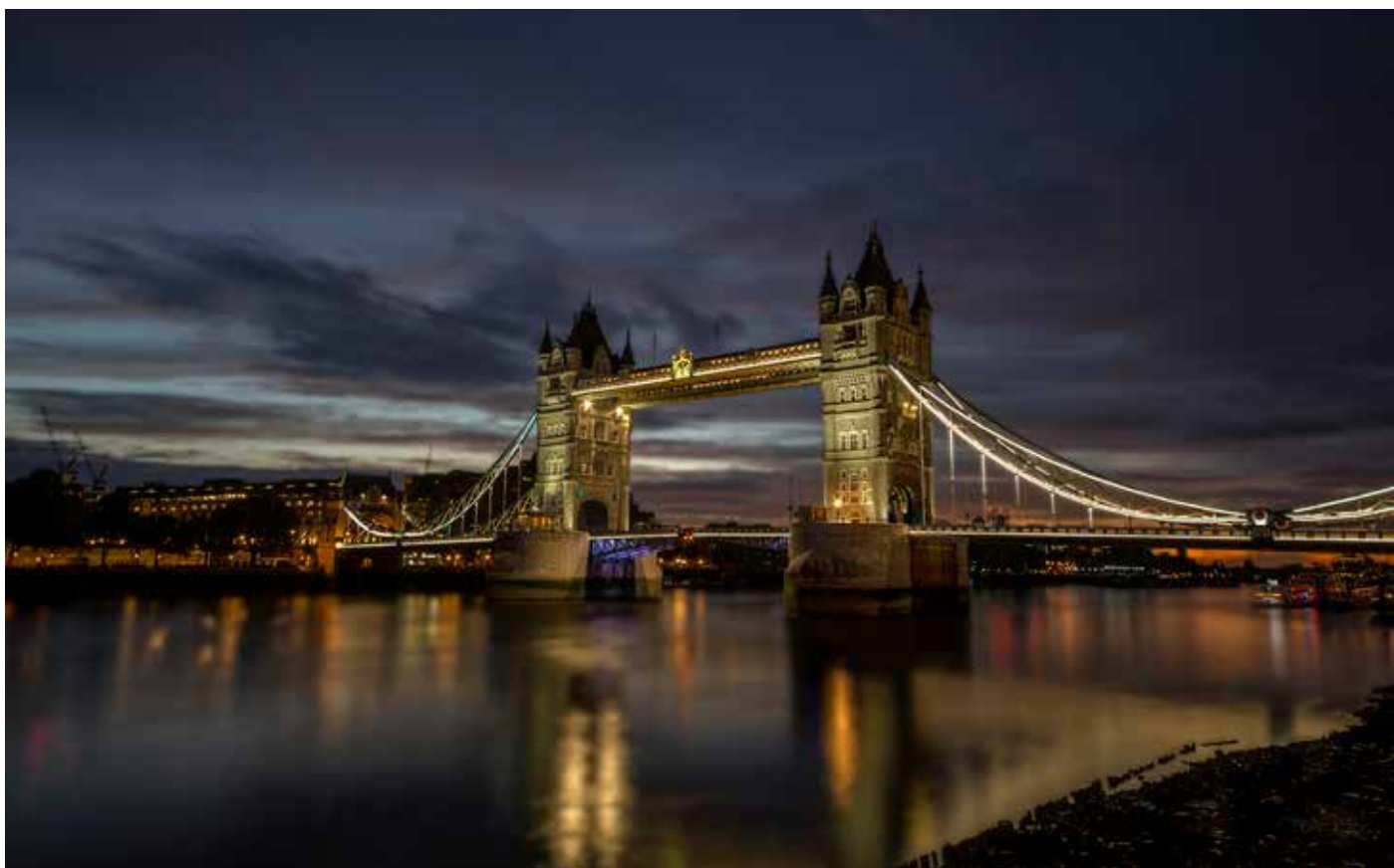
3 e prix - Vincent BONNEFILLE - Tower bridge - FRANCE
